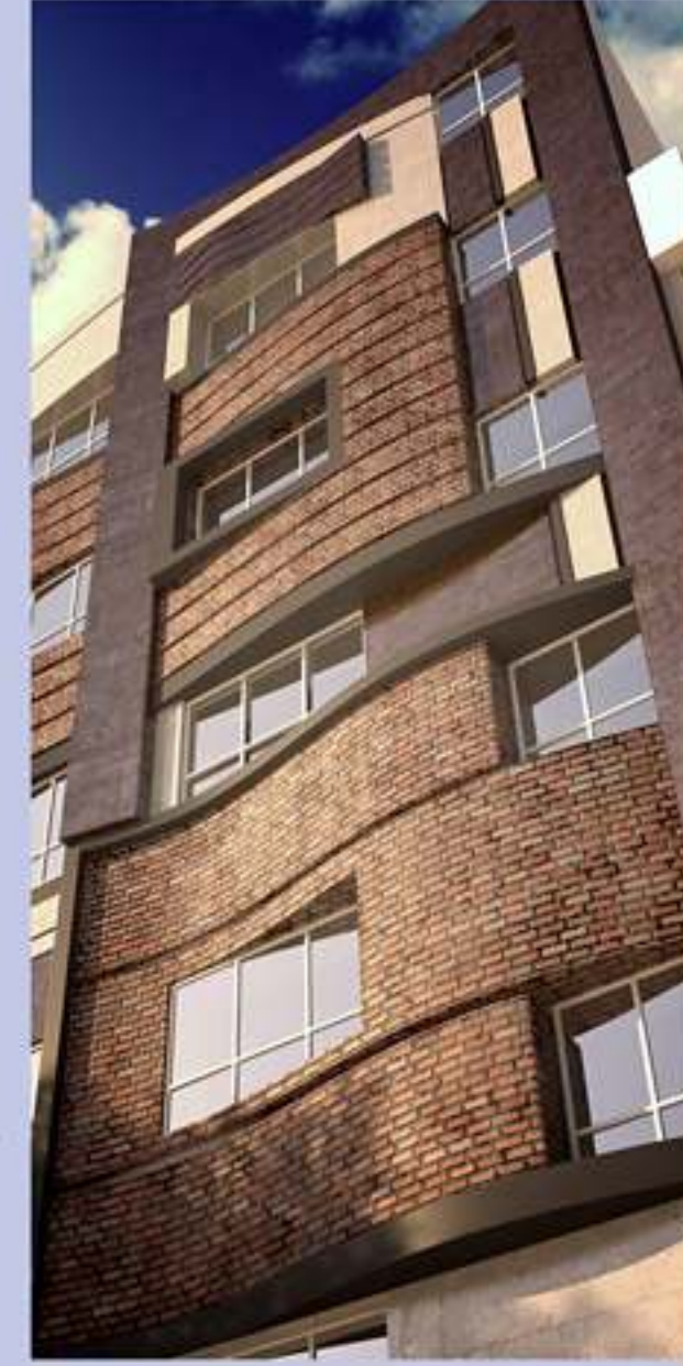
Modern Facade Design
